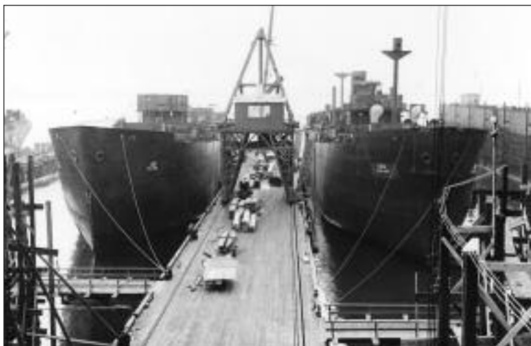
HULL 130 THE WINDERMERE PARK AND HULL 131 THE MOUNT BRUCE PARK BEING COMPLETED AT DOCKSIDE. (LAC PA187474)
